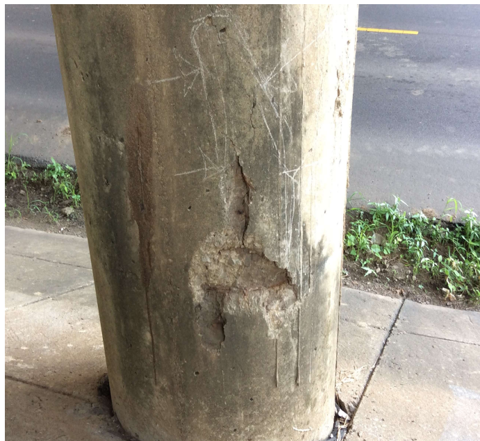
PHOTO 1 Description Bent 2 column 3, spalling with exposed reinforcing steel and delaminated areas.
