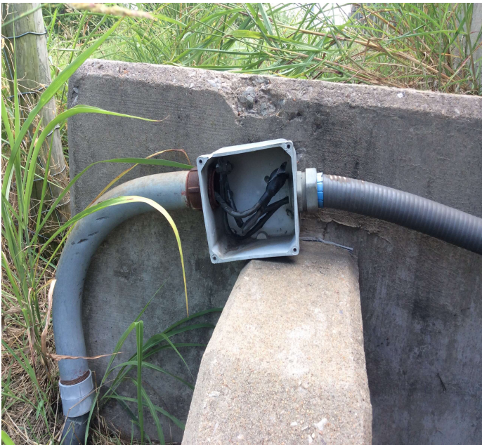
PHOTO 1 Description Bent 1 Right, utility box cover missing.
