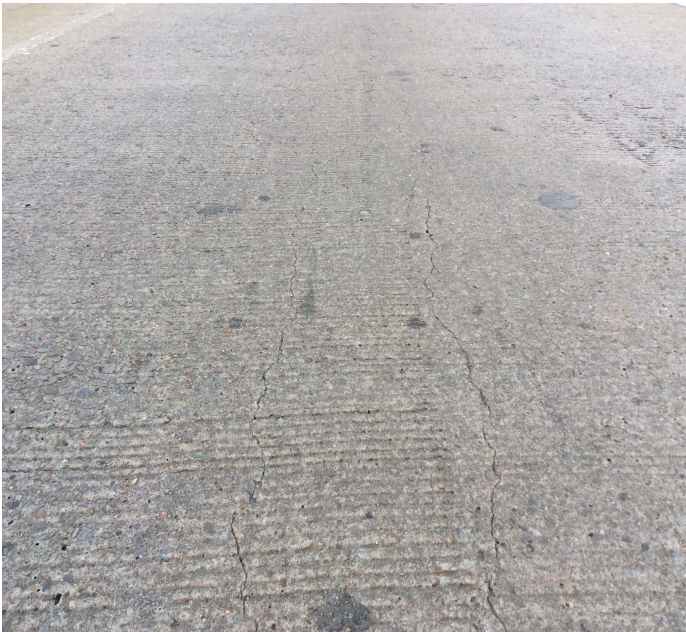
PHOTO 1 Description Full length longitudinal cracking in Right lane of span 3.
