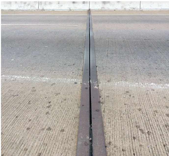
PHOTO 1 Description Bent 2 compression seal deteriorated.
