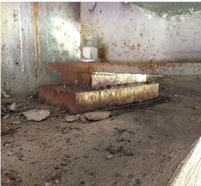
PHOTO 1 Description Bent 1 beam 6Active corrosion with flaking rust in bearing device.
