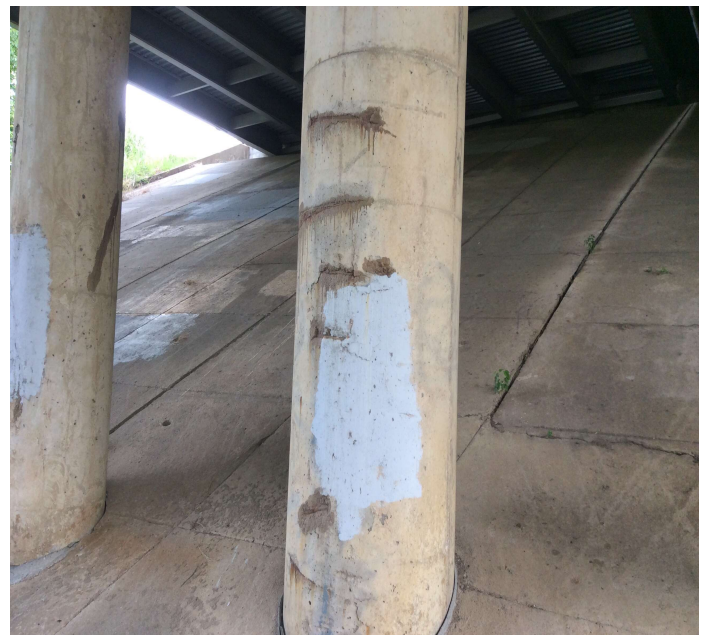
PHOTO 2 Description Bent 2 center column, spalling with exposed reinforcing steel.
