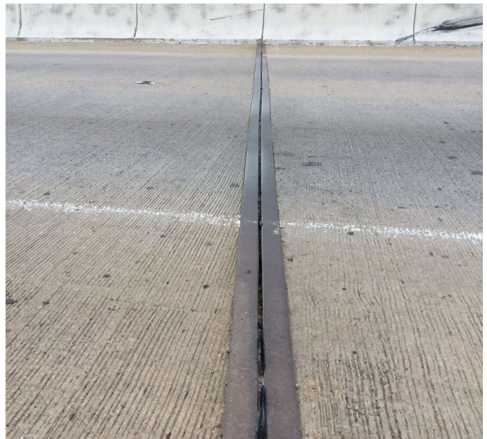
PHOTO 2 Description Bent 3 compression seal deteriorated.
