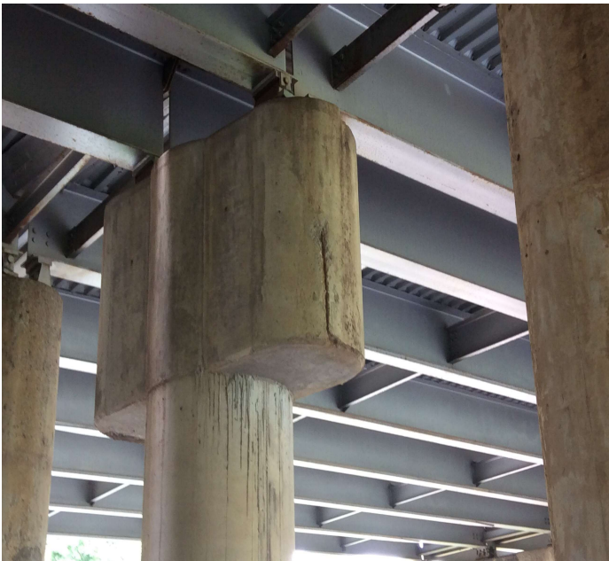
PHOTO 3 Description Bent 2 center cap under beam 1 has an area of spalling with exposed reinforcing steel.
